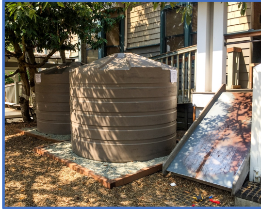
Building 2 Two 1,110-gallon Bushman cisterns with overflow to side sewer.
