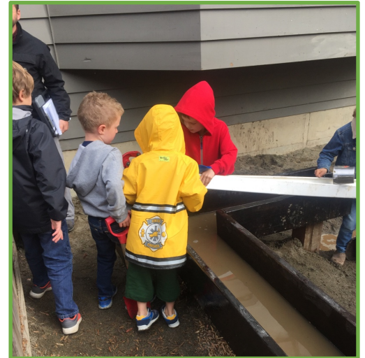
Children help with cistern installation.
