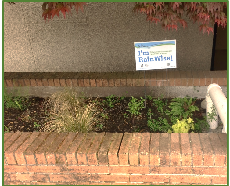
Rain Dog Designs installed a "vertical" rain garden in a planter box to capture water flow from the cisterns.
