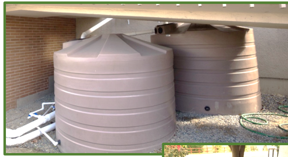
Cisterns under ramp.
